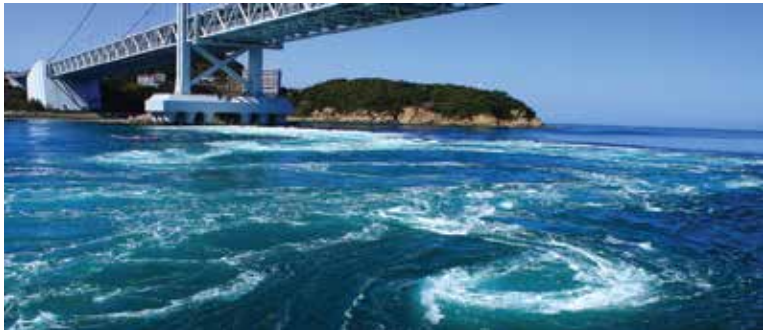
鸣门跨海大桥 Onaruto Bridge
